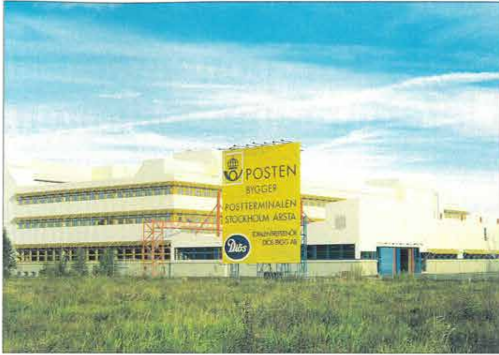
Postterminal in Stockholm Fertig 1990 40.000 m 2 Swedeck.
